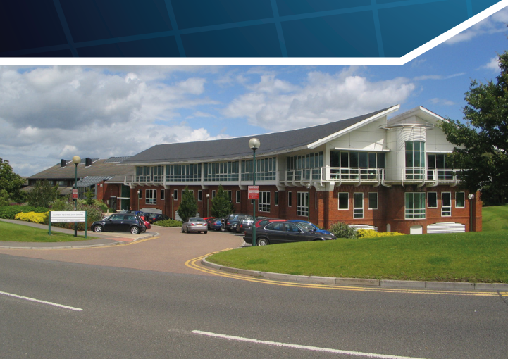
ANPR securing and monitoring business premises
